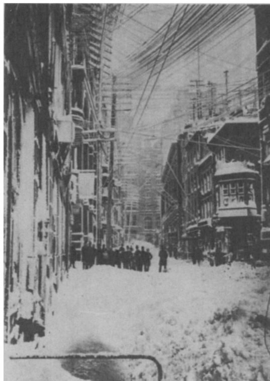
This view of New Street in New York City after a blizzard in 1888 shows the extensive telegraph and telephone network that served the city's financial district. Courtesy New York Stock Exchange Archives.
